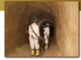
The existing sewer to be rehabilitated was approximately 80 years old and was located 20 ft. below ground. This project also included ten 4-foot-diameter manholes that were to be coated with SprayWall®, a structural coating.
